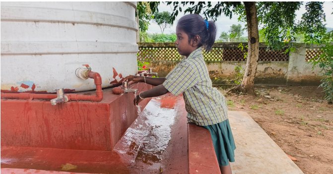
Toilets & handwash facilities are now clean and safe for students to access
